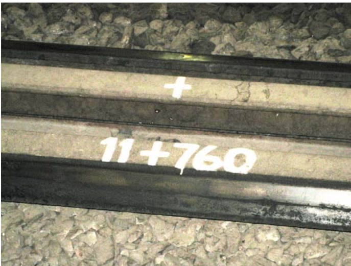
Mexico City, metro station (rail)
