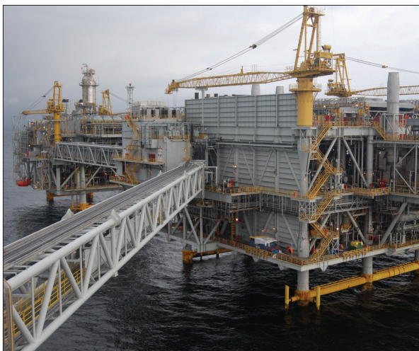
The East Area NGL II project includes extraction and fractionation facilities to recover natural gas liquids from gas gathered from the East Area fields offshore Nigeria.
