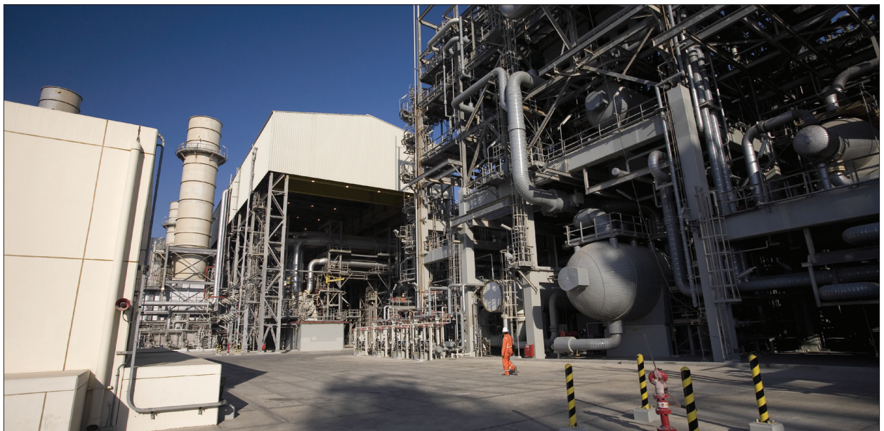
Qatargas II Train 4 is the world's largest LNG train with production capacity of 7.8 million tons per year. First LNG is expected in early 2009.
