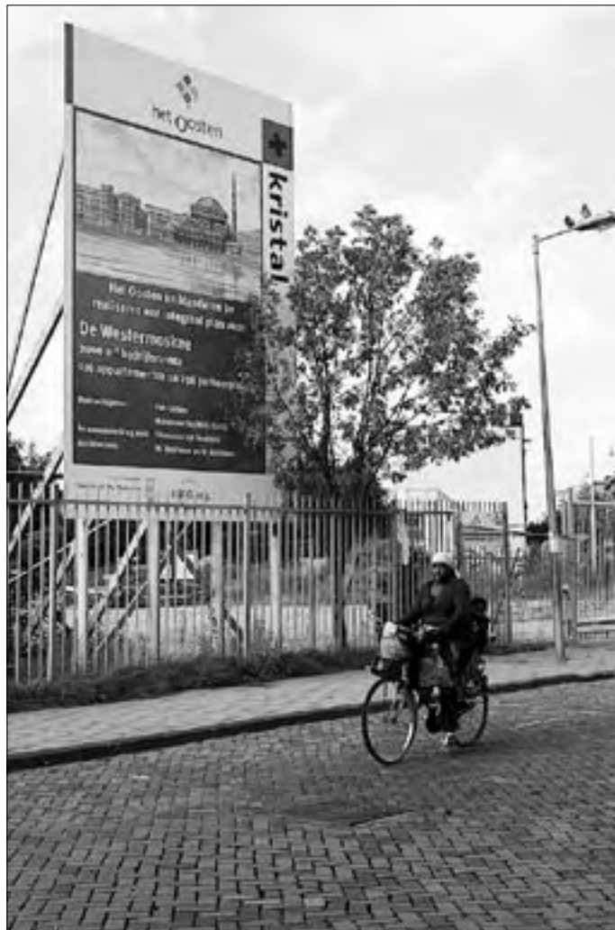
Construction site of the Western Mosque, Amsterdam
